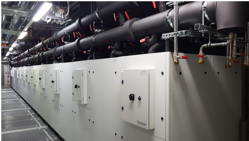
A Fahrenheit adsorption chiller converts the heat generated by the processors of the SuperMUC-NG supercomputer into cooling energy so that the computer uses it to cool itself.
